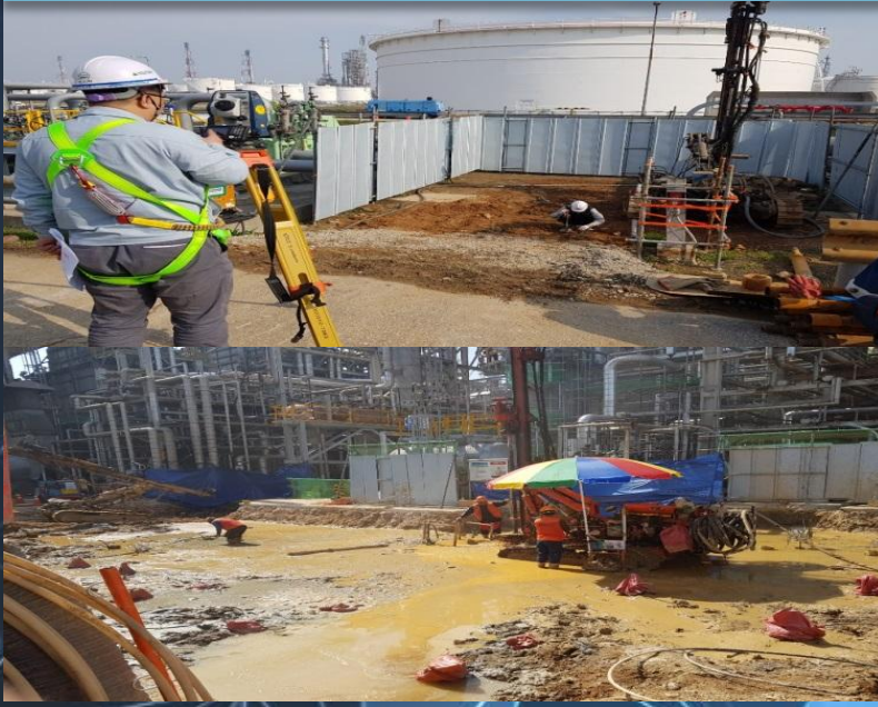
2018 HDO REVAMPING CDU PROJECT
