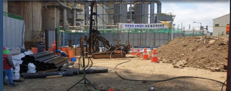
울산S-OIL #2 ARO H2 RICH GAS COMPRESSOR INSTALLATION
