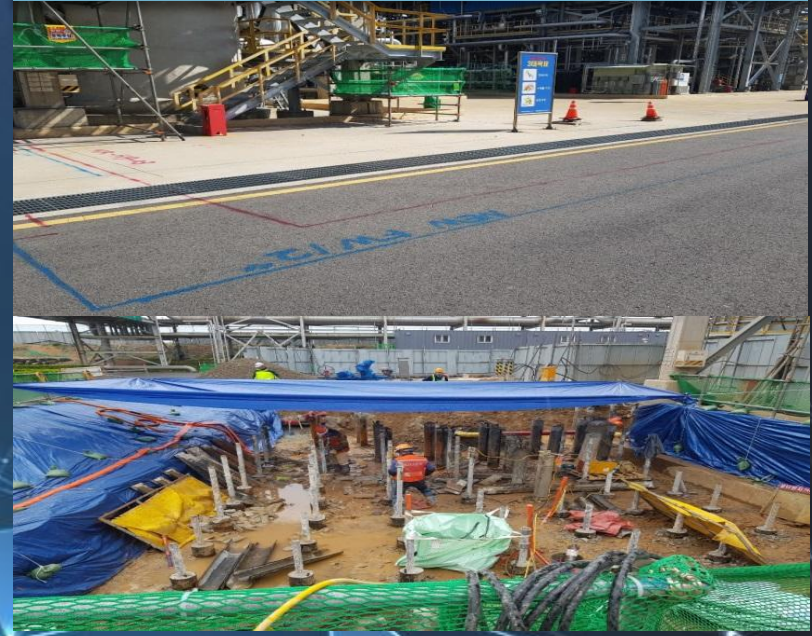
2018 HDO REVAMPING SRU HCR PROJECT
